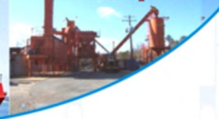
Simidia's Asphalt Plant
