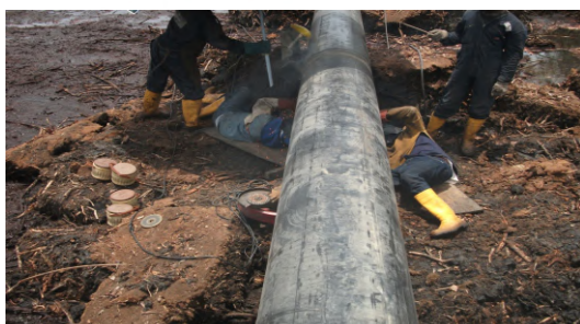
Construction of 24" x4km pipeline along Amukpe – Escravos pipeline route
