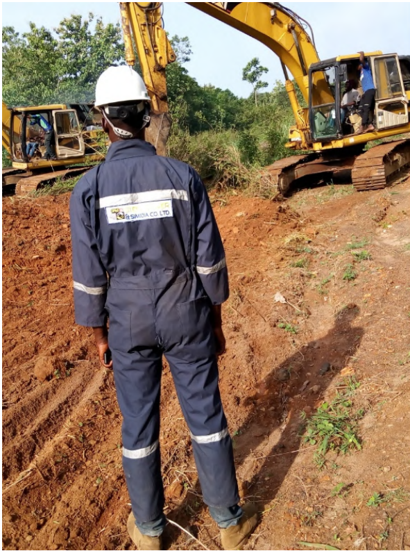
STEEL FLOWER & SIMIDIA EXCAVATORS CLEARING SWAMP AND PREPARING RIDGES
