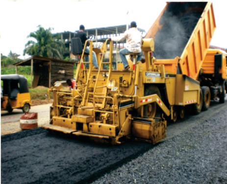
Priming and Laying of Asphalt @Olokoro-Itaja-Obuohia-Imuahia-Isicourt Road in Abia State
