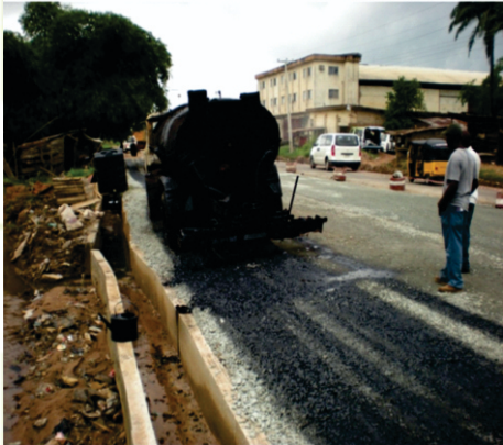
Priming and Laying of Asphalt @Olokoro-Itaja-Obuohia-Imuahia-Isicourt Road in Abia State
