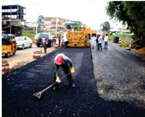
Priming and Laying of Asphalt @Olokoro-Itaja-Obuohia-Imuahia-Isicourt Road in Abia State
