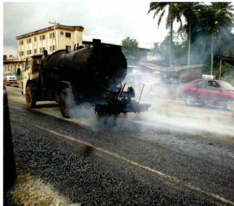
Priming and Laying of Asphalt @Olokoro-Itaja-Obuohia-Imuahia-Isicourt Road in Abia State
